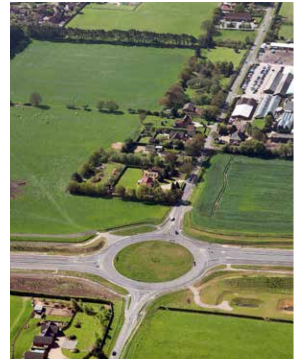
COMPLETED BROADLAND NORTHWAY JUNCTION
