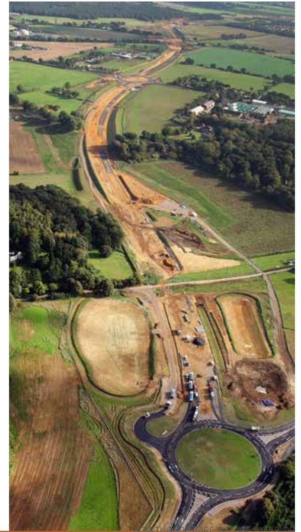
BROADLAND NORTHWAY UNDER CONSTRUCTION
