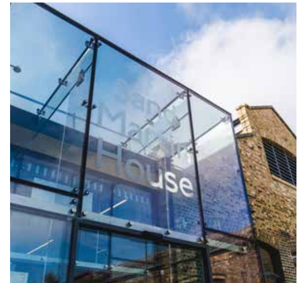
SAND MARTIN HOUSE EXTERIOR
