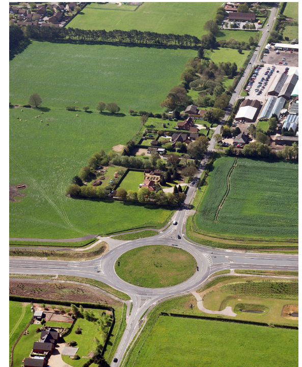
COMPLETED BROADLAND NORTHWAY JUNCTION
