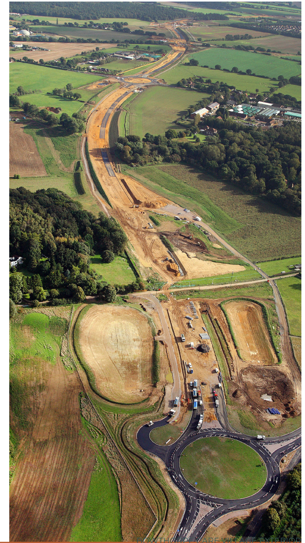
BROADLAND NORTHWAY UNDER CONSTRUCTION
