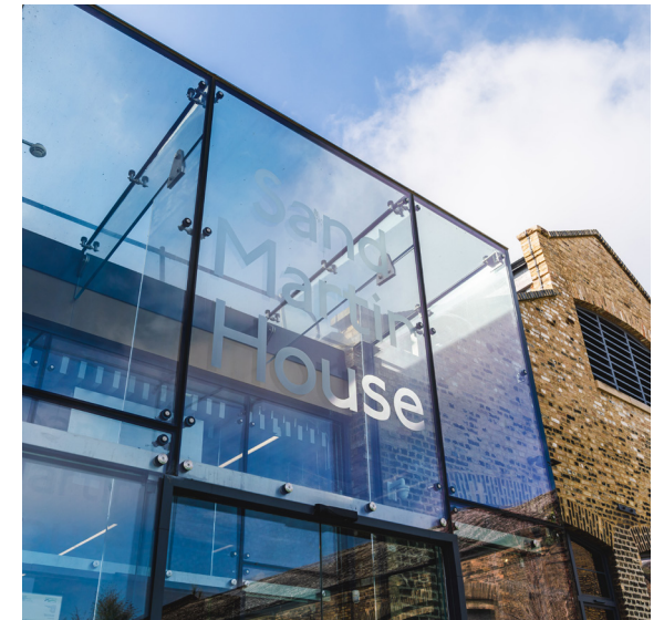
SAND MARTIN HOUSE EXTERIOR
