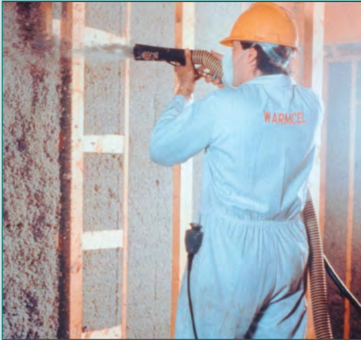
WARMCEL CELLULOSE INSULATION (RECYCLED NEWSPAPER) BEING SPRAY APPLIED PHOTO: EXCEL INDUSTRIES
