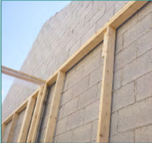
CONCRETE BLOCKWORK UNDER CONSTRUCTION PHOTOS.COM WEBSITE
