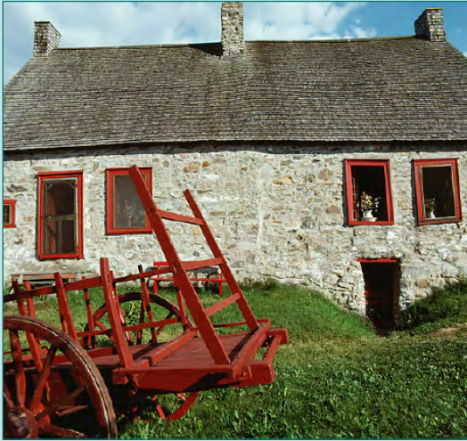
STONE IS USED EXTENSIVELY IN MANY HISTORIC CITIES AND UPLAND LOCATIONS PHOTOS.COM WEBSITE
