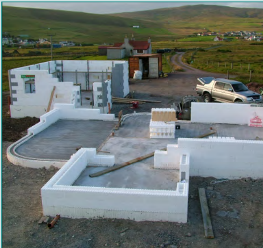
ICF HOUSE UNDER CONSTRUCTION PHOTO: THE CONCRETE SOCIETY
