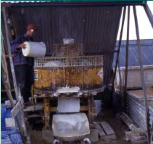
LIME MORTAR BEING MIXED PHOTO: JJ SHARPE
