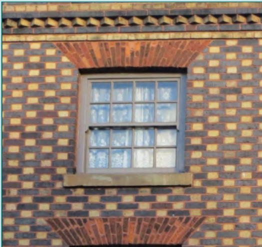
POLYCHROMATIC BRICKWORK IN CHESTER ALEX LIIVET FROM CHESTER, UNITED KINGDOM, CC0, VIA WIKIMEDIA COMMONS
