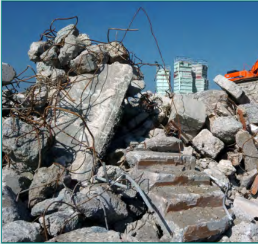
DEMOLISHED INSITU CONCRETE - RECYCLED AGGREGATE PHOTO: LA FARGE
