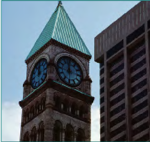
COPPER ROOFING PHOTOS.COM WEBSITE
