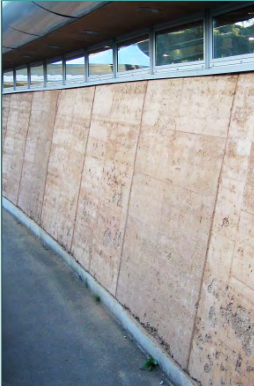
RAMMED EARTH VISITOR CENTRE AT THE EDEN PROJECT, UK PHOTO: ANDREW DUNN (WIKIMEDIA COMMONS)
