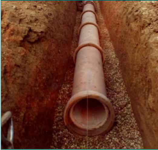
CLAY DRAINS BEING LAID PHOTO: NAYLOR DRAINAGE LTD
