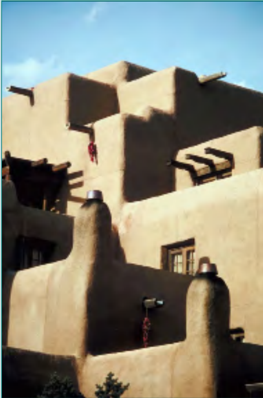
TRADITIONAL ADOBE BUILDINGS IN NEW MEXICO USA PHOTO: PHOTOS.COM WEBSITE
