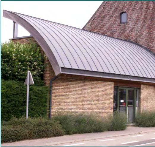
CURVED ZINC ROOFING PHOTO: KVDP (WIKIMEDIA COMMONS)
