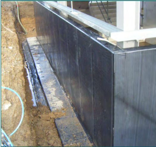
PEEL N STICK TANKING BITUMEN PHOTO: JO DENISON, STEPHEN GEORGE + PARTNERS
