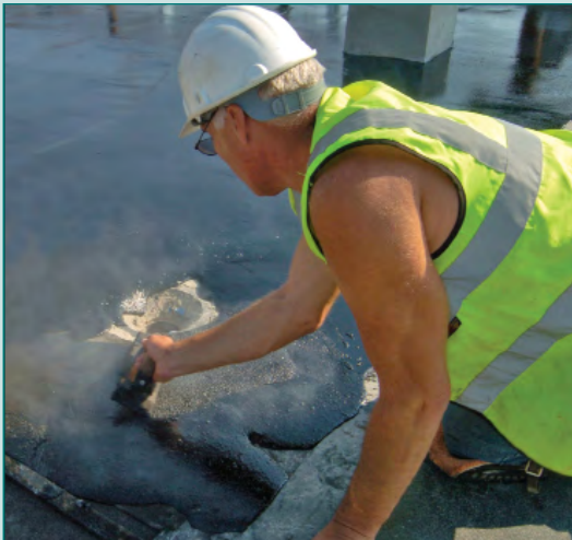
MASTIC ASPHALT BEING LAID PHOTO: MASTIC ASPHALT COUNCIL
