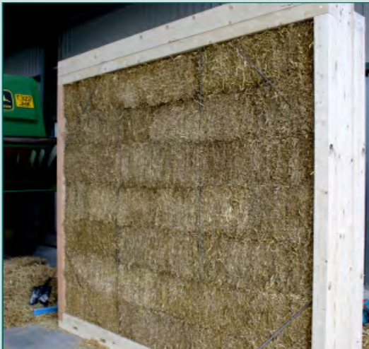
MODCELL PANELS UNDER CONSTRUCTION PHOTO: MODCELL (WWW.MODCELL.CO.UK)
