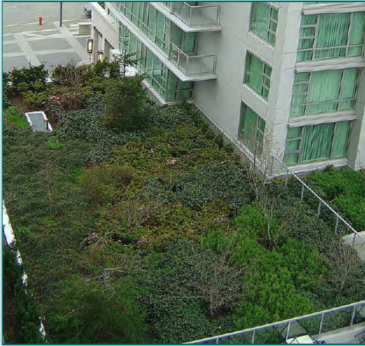
AN ESTABLISHED INTENSIVE GREEN ROOF. PHOTO: PNWRA (WIKIMEDIA COMMONS)
