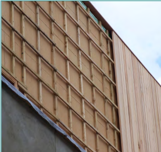
PAVACLAD SYSTEM UNDER CONSTRUCTION PHOTO: NATURAL BUILDING TECHNOLOGIES
