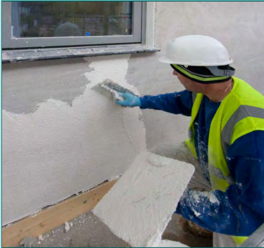
LIME RENDER BEING APPLIED PHOTO: COPYRIGHT © 2000-2009 LIME TECHNOLOGY LIMITED
