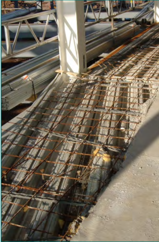
COMPOSITE STEEL-CONCRETE FLOORING BEING LAID. PHOTO: JOHN COOPER, STEPHEN GEORGE + PARTNERS
