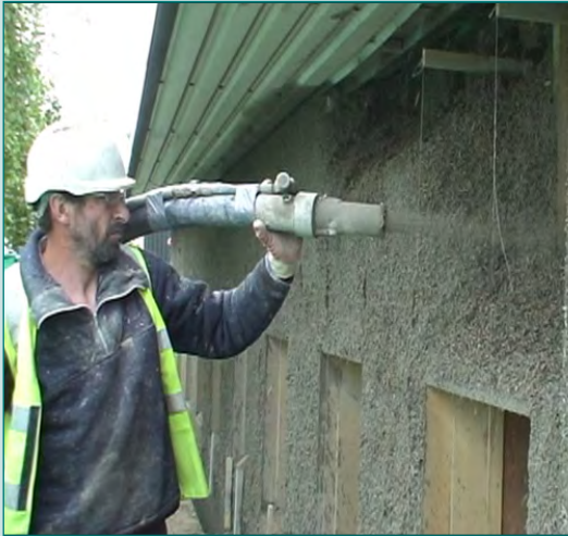
HEMCRETE BEING SPRAY APPLIED PHOTO: COPYRIGHT © 2000-2009 LIME TECHNOLOGY LIMITED)
