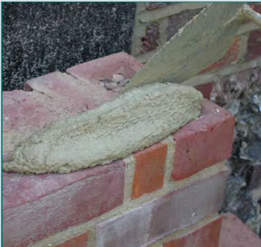
LIME MORTAR BEING APPLIED PHOTO: COPYRIGHT © 2000-2009 LIME TECHNOLOGY LIMITED
